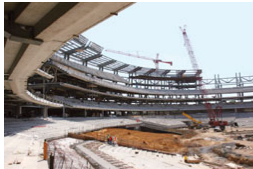
Thornton Tomasetti, Inc. Job cut into discrete design and construction sequences, beginning on right field side, to save six months.
